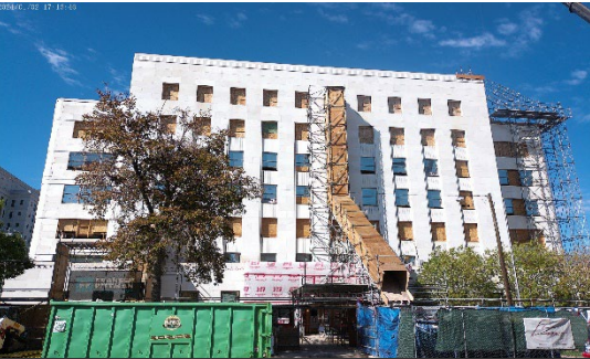
COLORADO STATE CAPITAL ANNEX BUILDING
