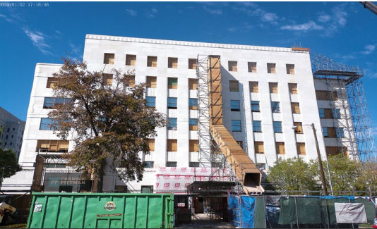
COLORADO STATE CAPITAL ANNEX BUILDING
